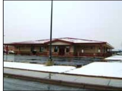
Illustration 3-1 Office Building along HWY 380
