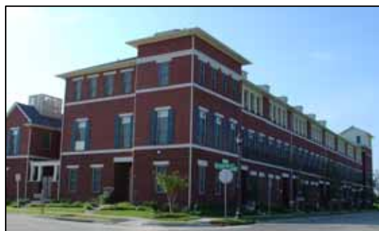
Illustration 4-5 An Example of Horizontal Mixed Use Design Concept (Residential building in a mixed use development)
