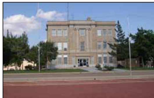
Illustration 6-8 Terry County Courthouse
