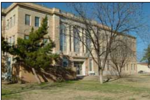
Illustration 6-7 Terry County Courthouse
